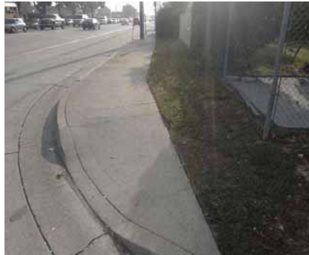
Curb Ramp : Bottom Landing Slope
