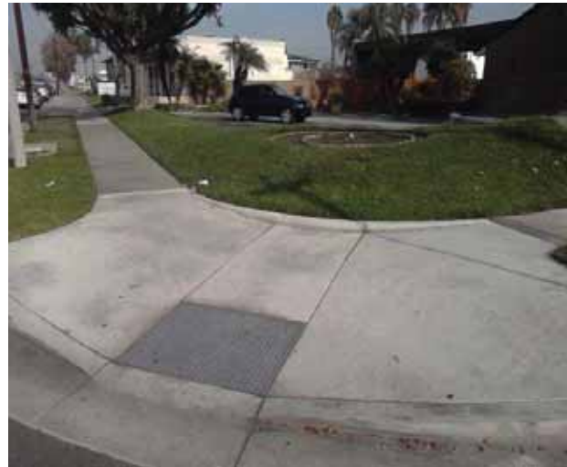
Curb Ramp : Bottom Landing Slope
