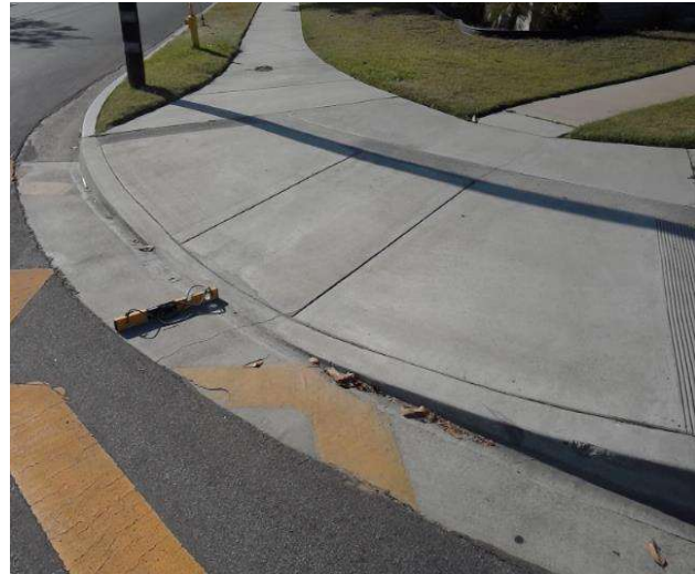
Curb Ramp : Bottom Landing Slope
