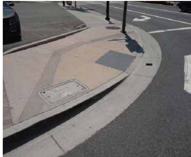
Curb Ramp : Bottom Landing Slope
