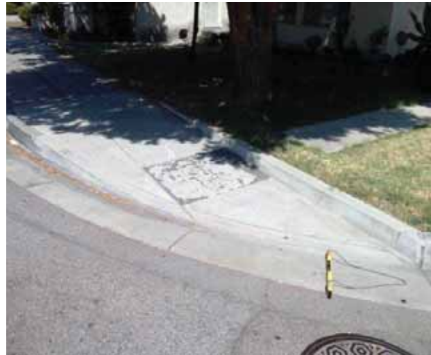
Curb Ramp , Landings and Transitions : Top Landing Change in Level - Curb Ramps
