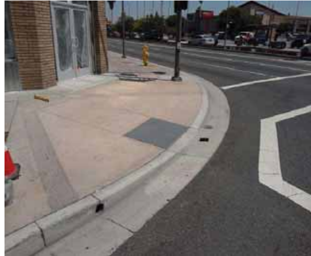
Curb Ramp : Bottom Landing Slope
