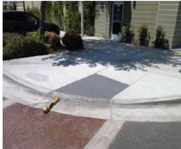
Curb Ramp : Bottom Landing Slope
