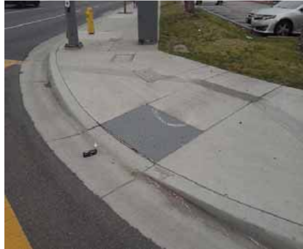
Curb Ramp : Bottom Landing Slope
