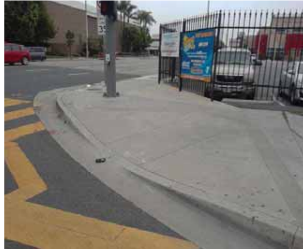
Curb Ramp : Bottom Landing Slope
