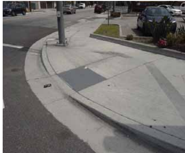
Curb Ramp : Bottom Landing Slope
