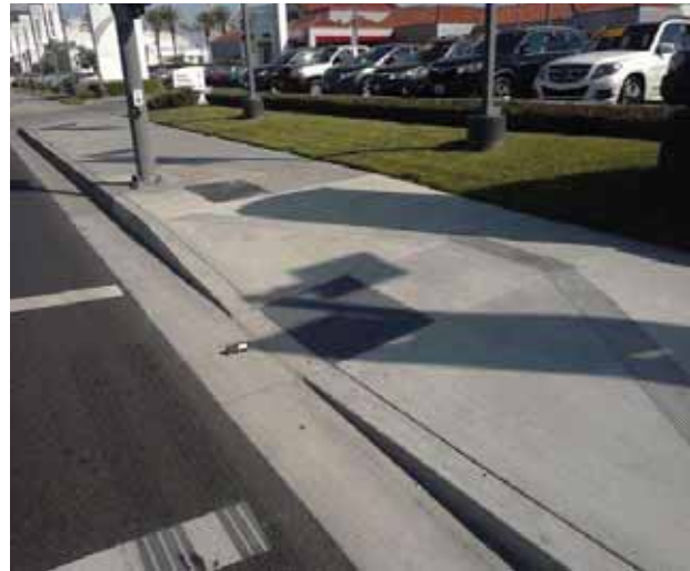
Curb Ramp : Bottom Landing Slope
