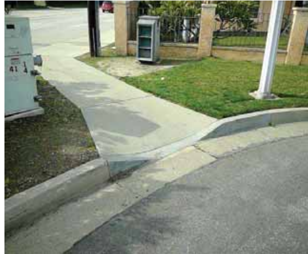
Curb Ramp , Landings And Transitions : Bottom Landing Change in Level due to Overlayment
