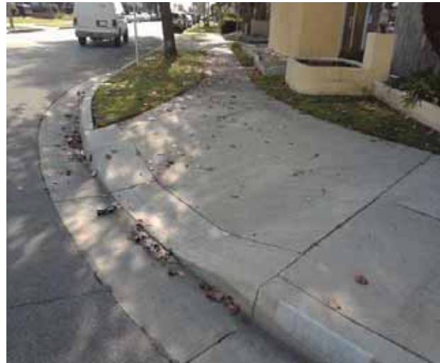
Curb Ramp : Bottom Landing Slope
