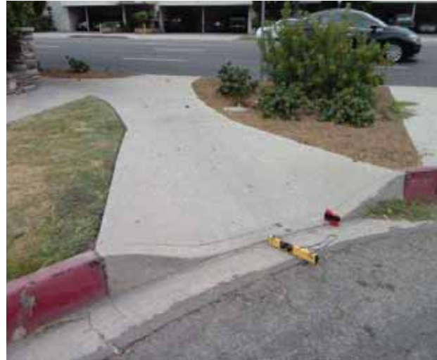
Curb Ramp : Bottom Landing Slope
