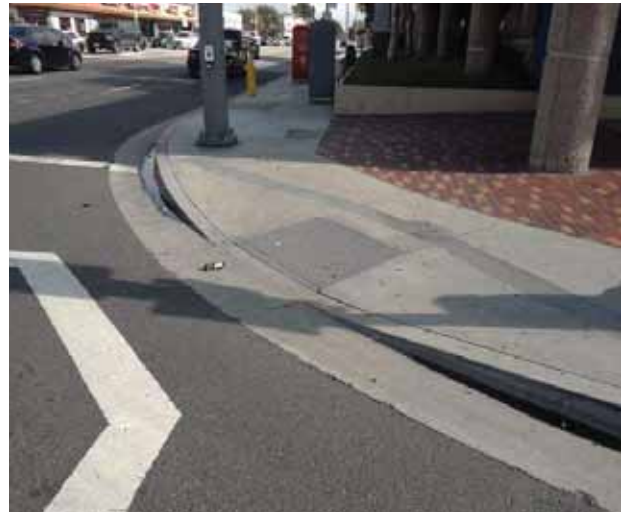
Curb Ramp : Bottom Landing Slope
