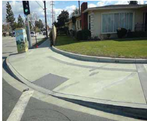
Curb Ramp : Bottom Landing Slope
