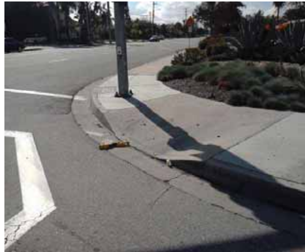
Curb Ramp : Bottom Landing Slope
