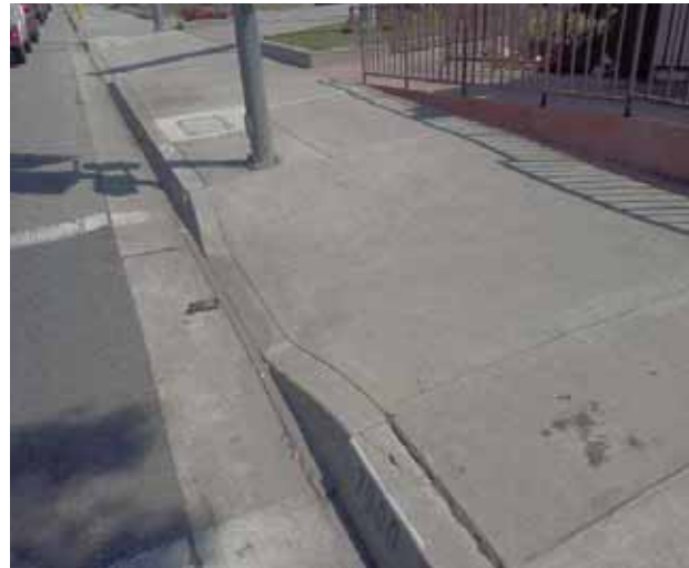
Curb Ramp : Bottom Landing Slope
