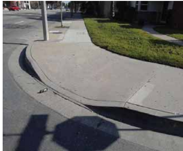
Curb Ramp : Bottom Landing Slope
