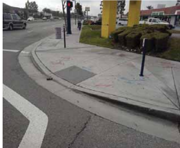
Curb Ramp : Bottom Landing Slope
