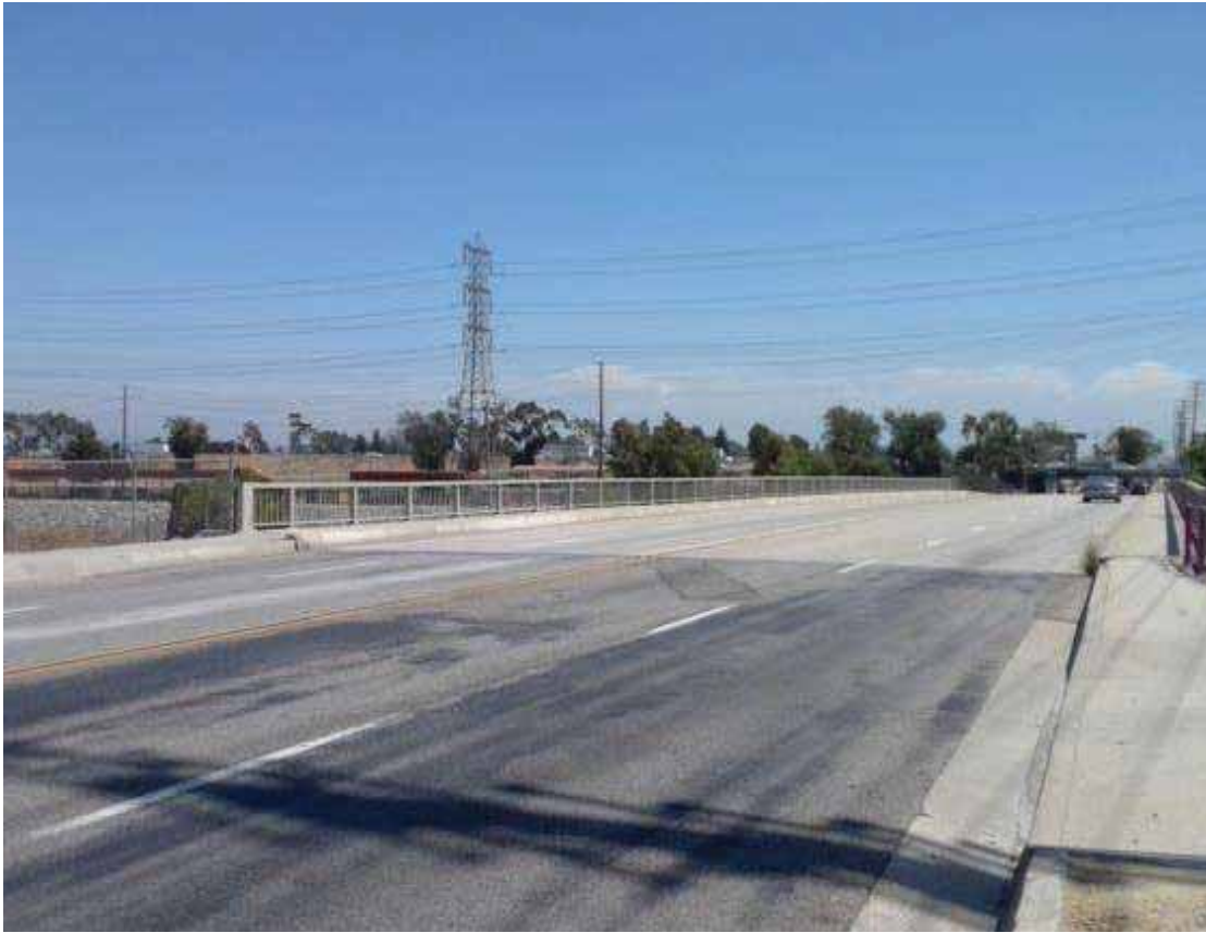
Florence Avenue Bridge Over San Gabriel River
