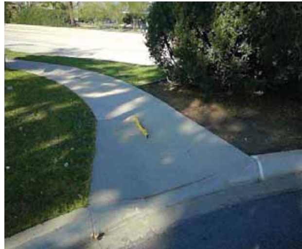
Curb Ramp : Bottom Landing Slope
