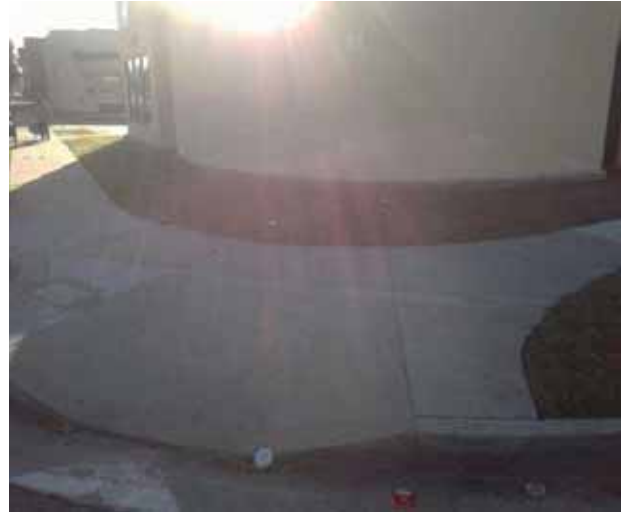
Curb Ramp : Bottom Landing Slope
