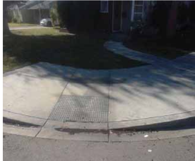
Curb Ramp : Bottom Landing Slope
