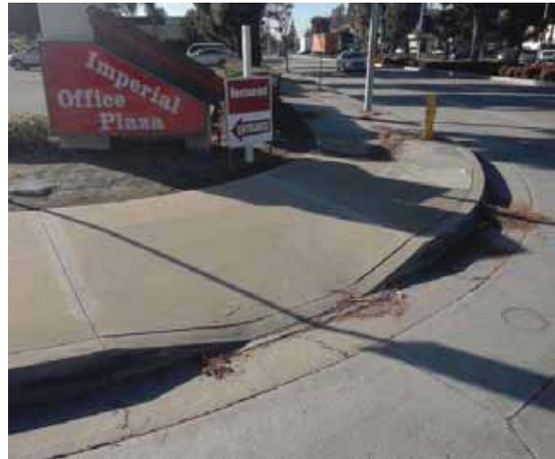
Curb Ramp : Bottom Landing Slope
