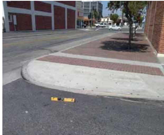
Curb Ramp : Bottom Landing Slope
