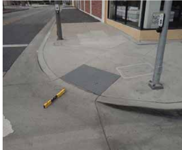
Curb Ramp : Bottom Landing Slope
