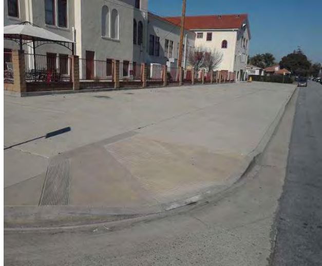
Curb Ramp : Bottom Landing Slope
