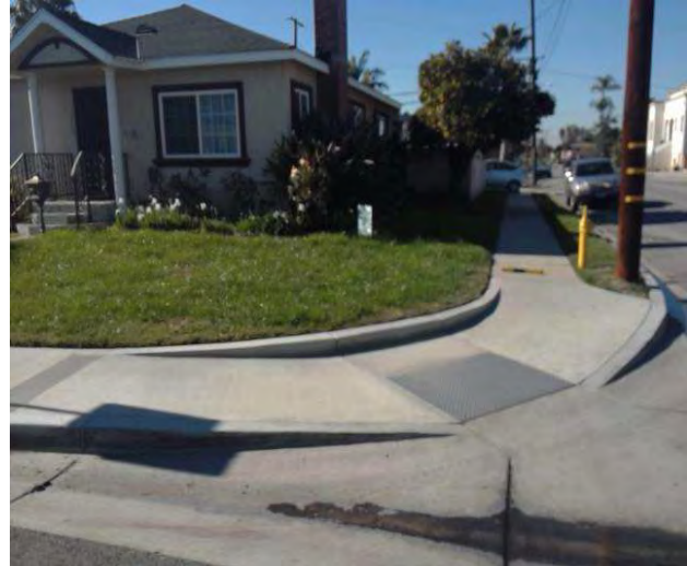
Curb Ramp , Landings and Transitions : Top Landing Right Side Change in Level - Curb Ramps
